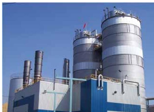
The anaerobic effluent treatment reactor at Témiscaming produces bio-gas for the mill's pulp drying process
